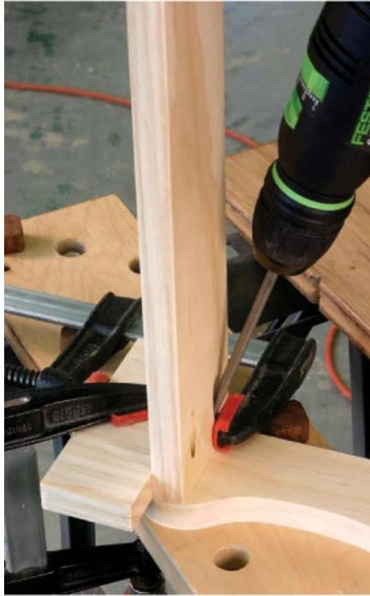
An offcut makes a handy clamping block to help you keep the shelves in place as you drive the pocket screws.
