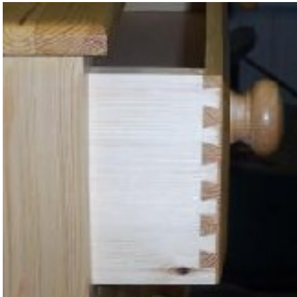
Half-lapped dovetail
