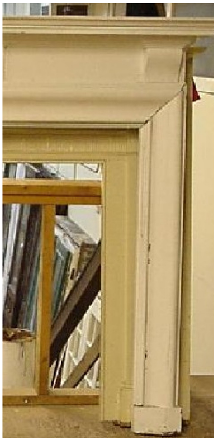
Figure 34: An antique mantel that shows shrinkage of the wood in the mitered joints
