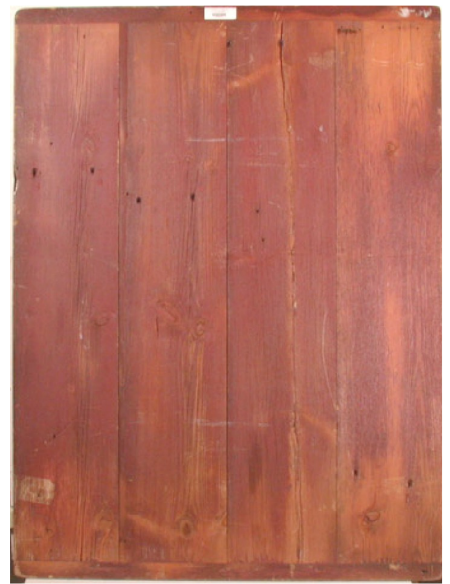
Figure 32: Panel split from restraint of glued lumber edge band
