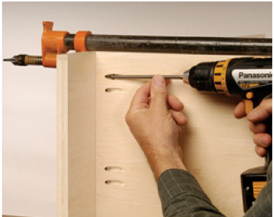
Pocket hole to reinforce a butt joint
